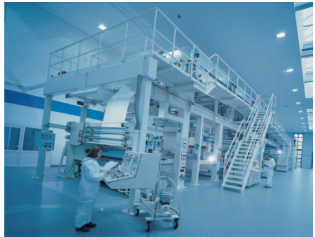
Modern production facility for the production of our innovative products
